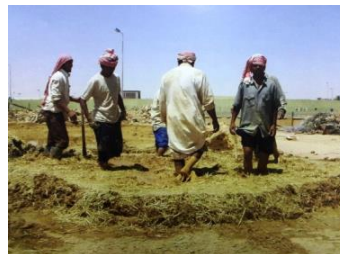
Figure (65) The mixing up process by the mixers (mulabineen) feet
