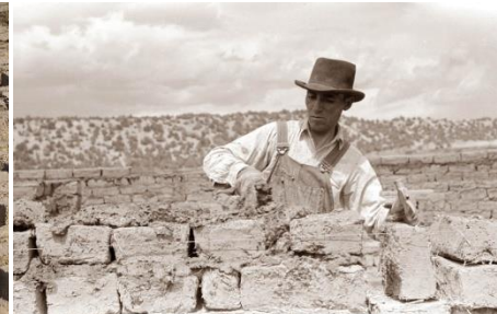
Figure (26) Adobe blocks in use by an expert
