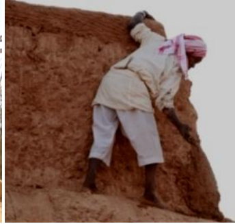
Figure (62) Cob (labin) construction technique using the layers (oroag) method
