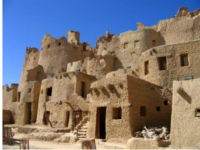
Figure (1) Fortified buildings made of karsheef mud buildings built by Siwan Berbers
