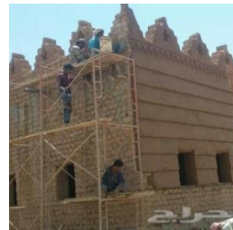
Figure (70) Building and finishing imitation of traditional mud buildings
