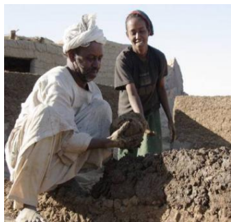
Figure (40) Cob as a building material used in building by house owners
