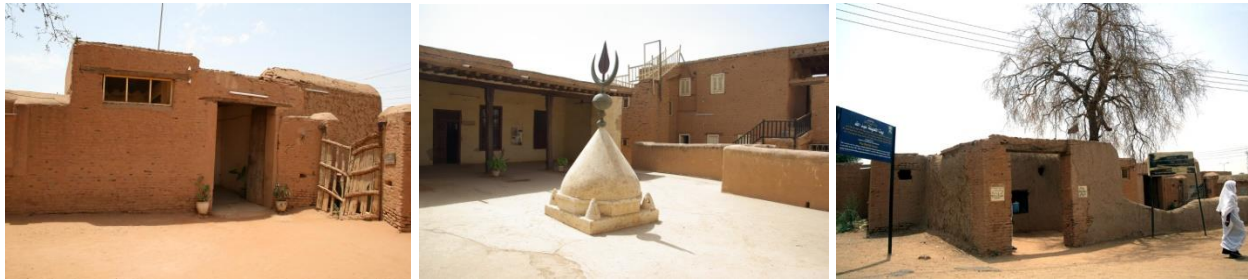
Figure (55) The Khaleefa's house, a significant historical museum, built out of cob
