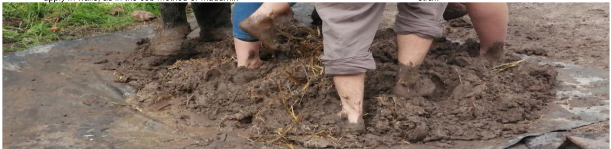
Figure (33) Adobe preparation by mixing the soil with water in the addition of hay or chopped straw well mixed by foot
