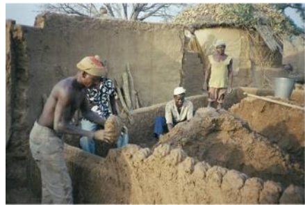
Figure (20) large blocks of lumps laid neatly side by side
