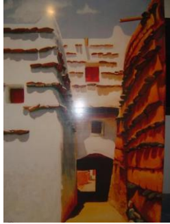
Figure (61) Projecting course of flat coral stones
