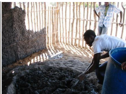
Figure (35) Fermentation resulting from mixing silt, hay and cow dung
