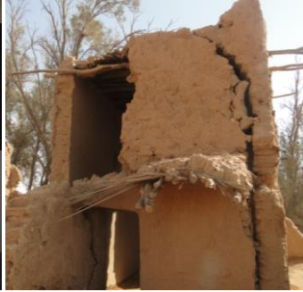
Figure (62) Cob (labin) construction technique using the layers (oroag) method
