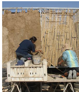
Figure (27), (28) and (29) showing different techniques of working on a wattle and daub walls
