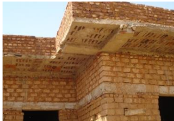
Figure (45) The vault roofing system of the researcher's adobe house
