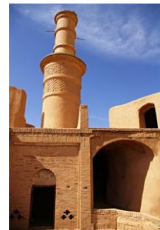
Figure (6) Old adobe minaret in Kharanagh village, Iran
