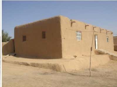
Figure (38) In old areas in almost all towns of the Sudan, people built by cob
