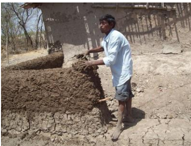
Figure (18) A cob wall under construction
