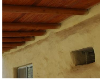
Figure (42) Cob's timber roofing system
