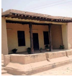
Figure (42) Cob's timber roofing system
