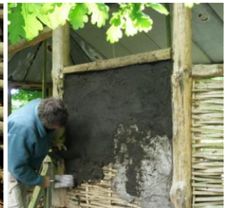
Figure (27), (28) and (29) showing different techniques of working on a wattle and daub walls
