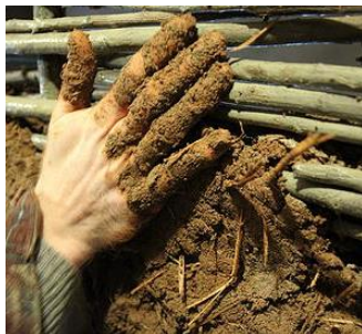
Figure (27), (28) and (29) showing different techniques of working on a wattle and daub walls
