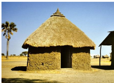
Figure (52) Wattle and daub house construction in the Doleib Hill, Sudan, 1977
