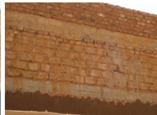
Figure (46) The wall plastered (dark) on interwoven wire mesh of iron
