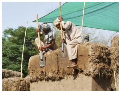
Figure (19) Rows of cobs of mud laid neatly on top of each other and pressed together
