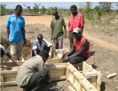
Figure (21) Making the formwork of rammed earth walls
