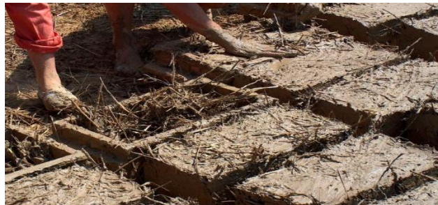
Figure (32) Molds of adobe blocks containing hay or chopped straw
